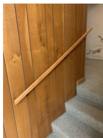
New handrail on small landing
